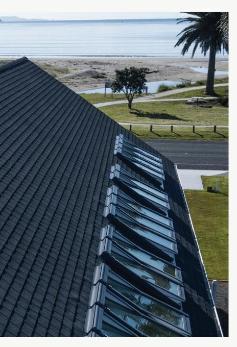
The architect for this project harnessed natural light beaming down from the roof to illuminate the upper level of the home, as well as penetrate down to the lower level. This was achieved with 36 VELUX skylights. In the architectural world, natural light is always preferable to artificial light.
